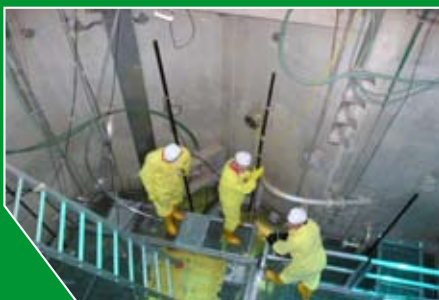
Working on the temporary grid in the vessel.
