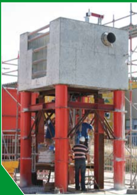
Drilling in the mock up
