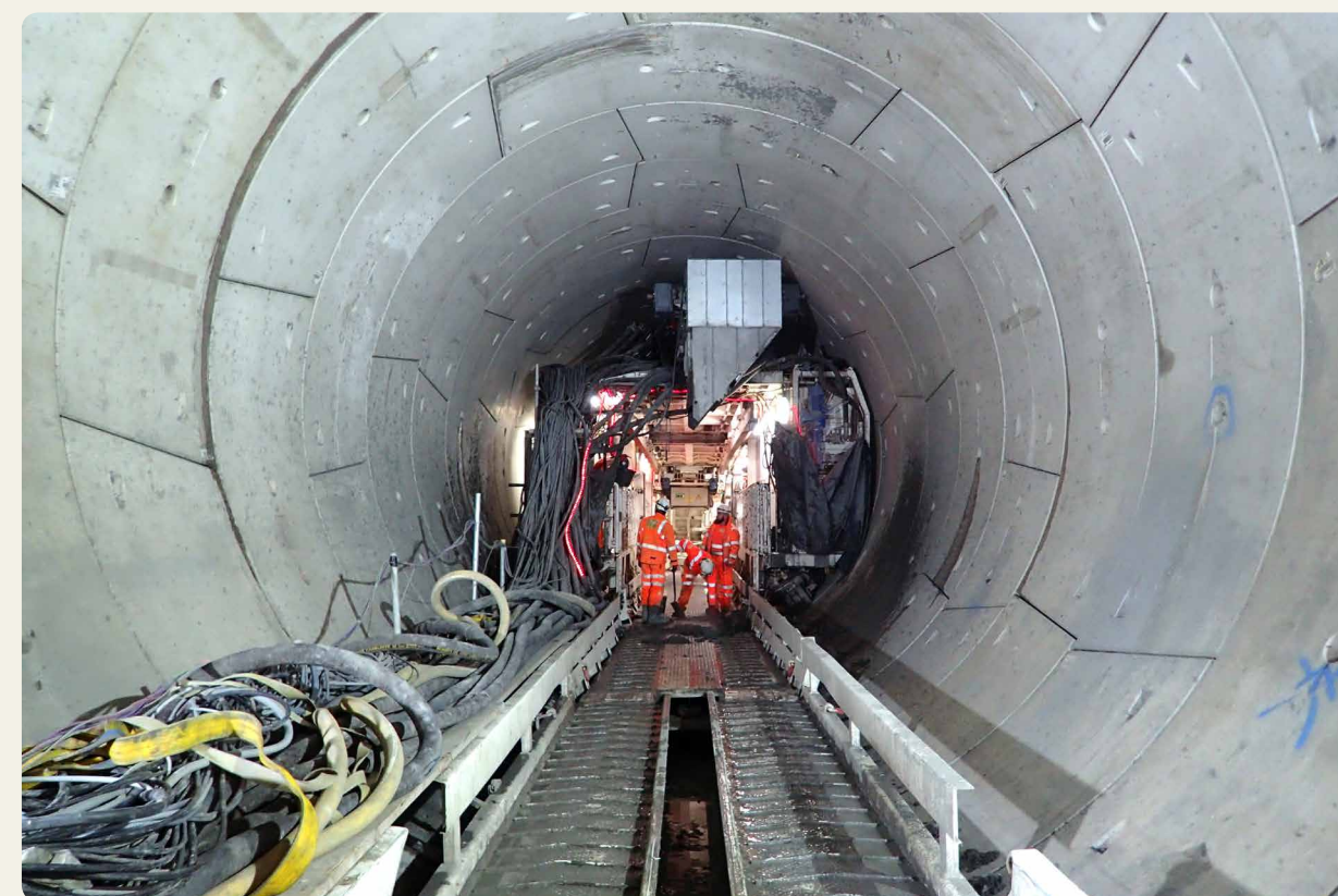
Figure 15. Tunnelling for the outfall and intake systems at Hinkley Point C, showing prefabricated concrete liner segments. (Moore, 2019)
